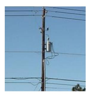
Distribution Lines send the electricity to smaller transformers which further step down the voltage on its way to the customer.
