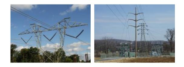
• Transmission lines connect to substations with transformers which step down the voltage.
